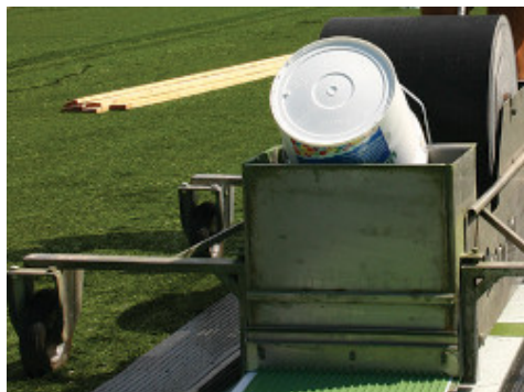
Fig. 2 - Application of Ultrabond Turf 2 Stars Pro using a continuous and controlled spreading system
